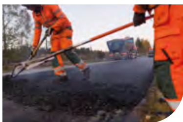
Construction materials and asphalt
